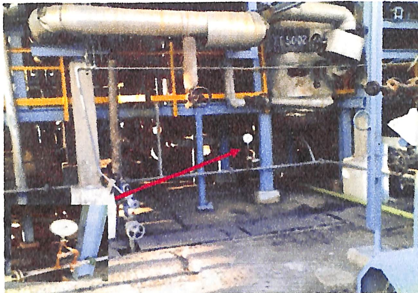
Fig6: Reboiler draining with Nitrogen & Demineralized water flushing (TT- 5002/TT-5003 & TT-1016) after implementation of the COSHH project.
