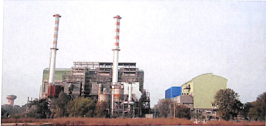
Figure 13 : Incineration plant at Timarpur- Okhla, New Delhi
