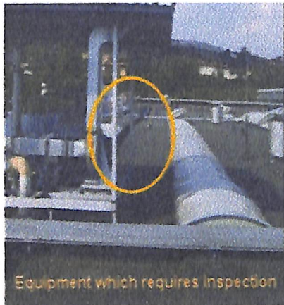
The inspection area is 0.6 m from a skylight consisting of Plexiglas.
