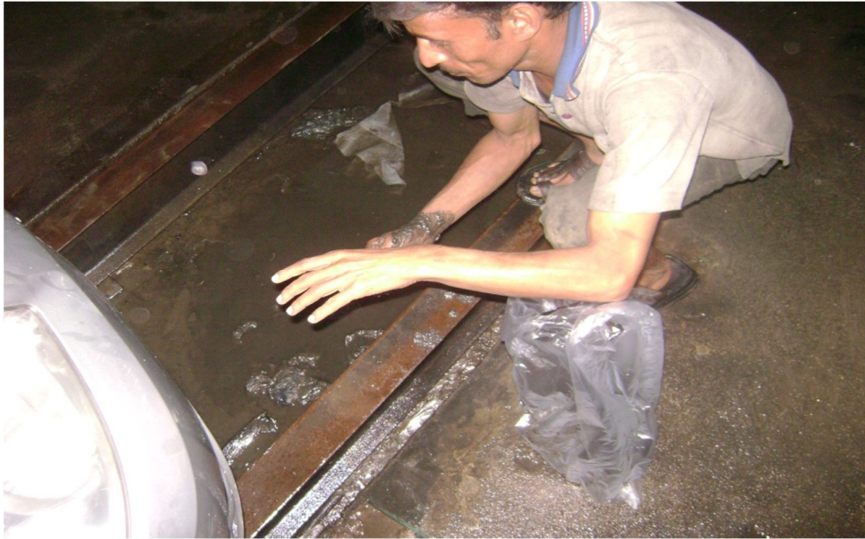
Figure 1.4 Discharge of waste water
