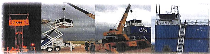
Photo 4: Relocation of Kalemie ATC tower/MONUSCO ASU
