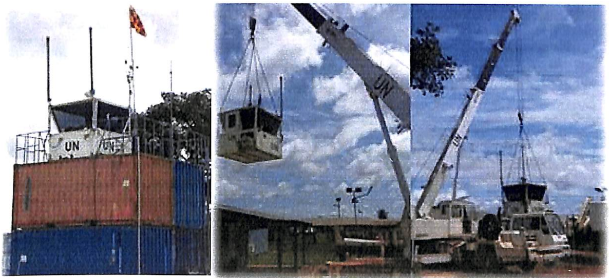
Photo 9: Dungu, Erection of new ATC tower MONUSCO Aviation ASU/2016
