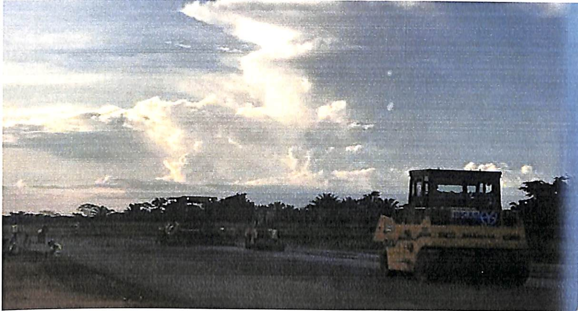
Photo6: Beni Runway Asphaltting ASU/MONUSCO AVIATION
