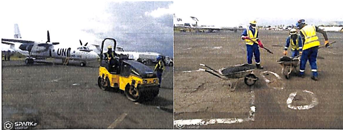
Fig 14: Goma Airport maintenance/AU/Spark
