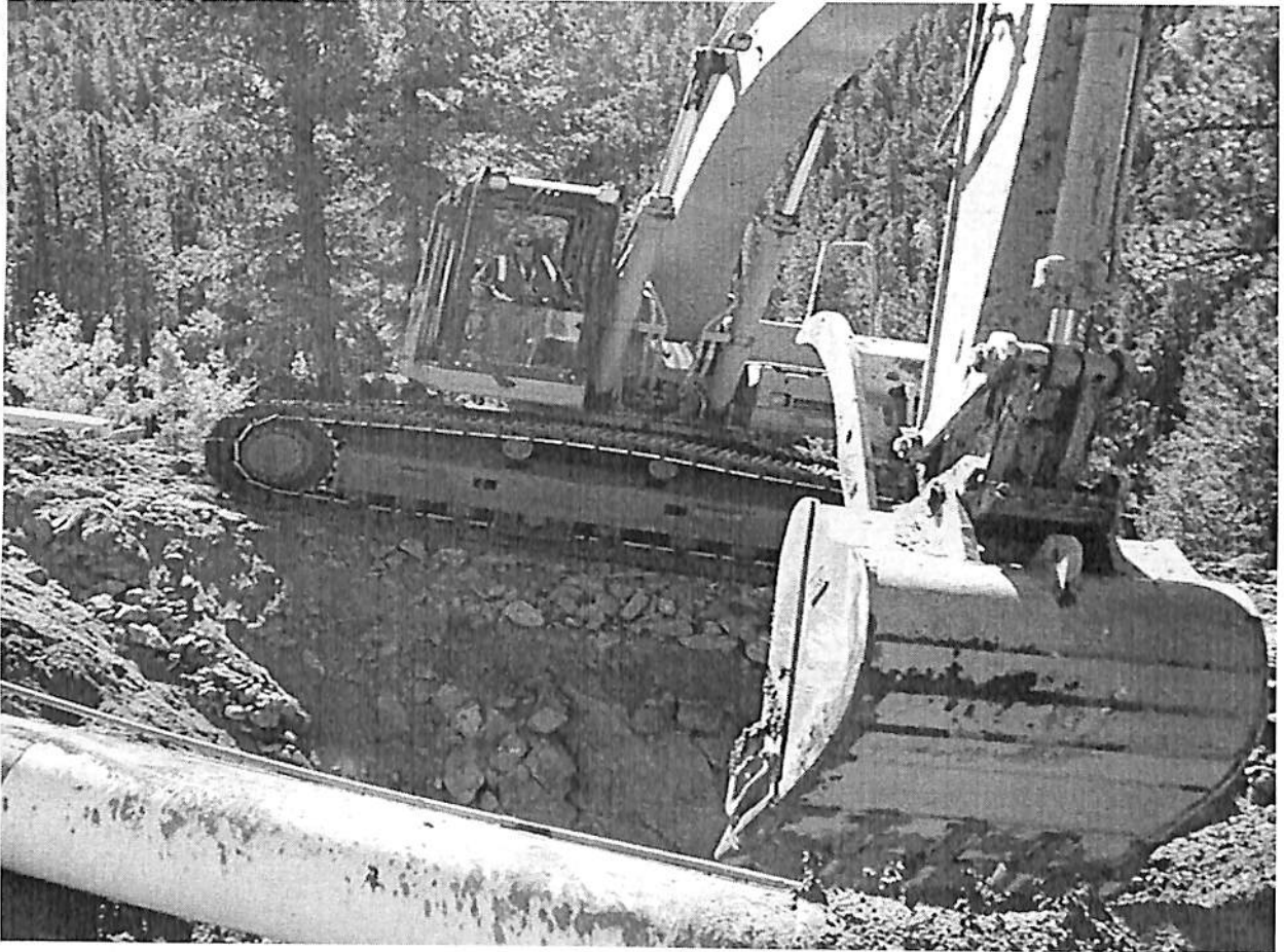
Backhoe trenching at site
