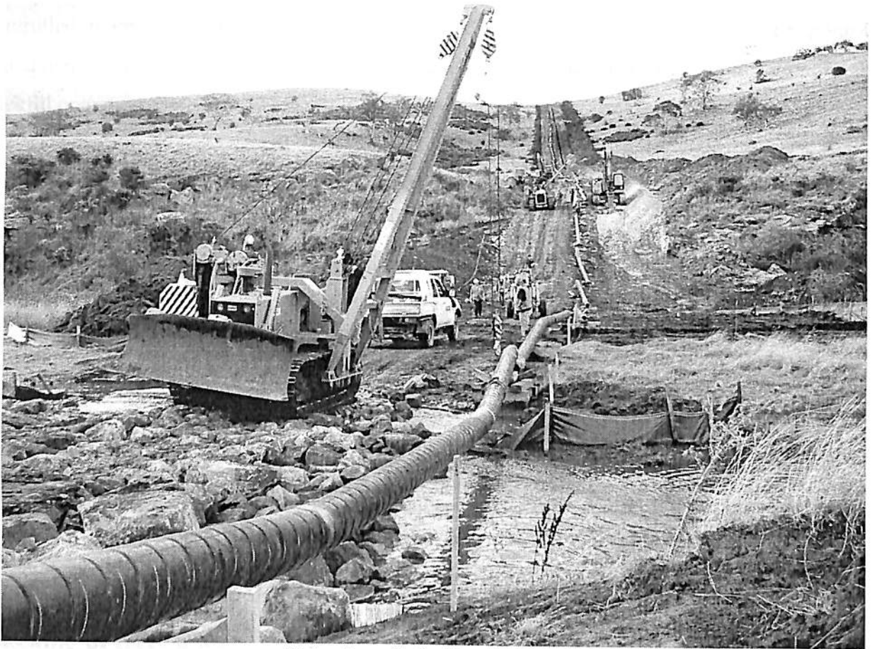
Stringing of pipeline
