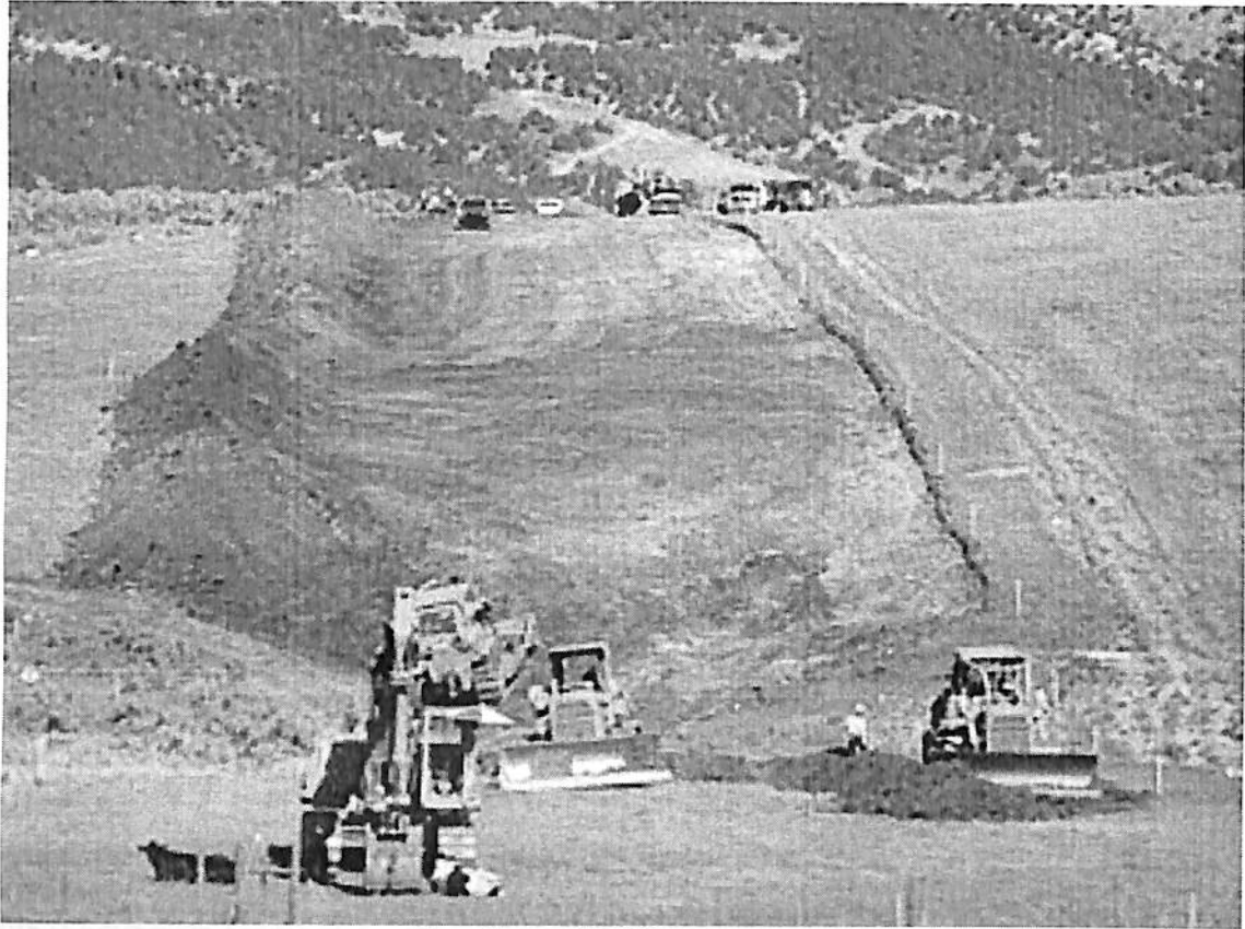
Grading of ROU
