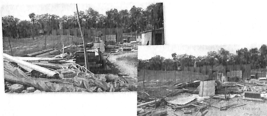
Figure 3.11 Site Photograph for Criterion 24
