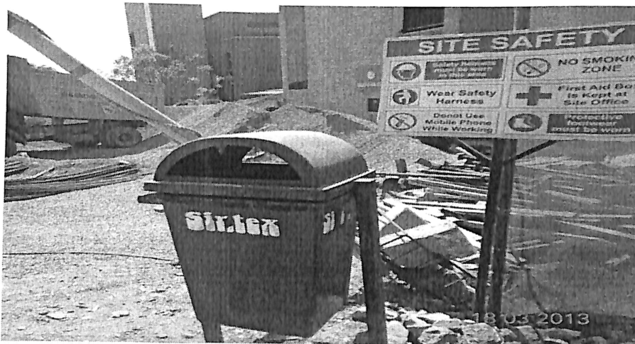
Figure 3.10 Site Photograph for Criterion 23
