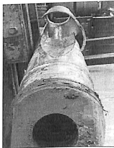
Figure 9.6 The swage diverter after removal from the well. Note the slot on the left that orients against the formed metal junction profile and ensures proper alignment of the diverter in order to provide entry into leg #1.
