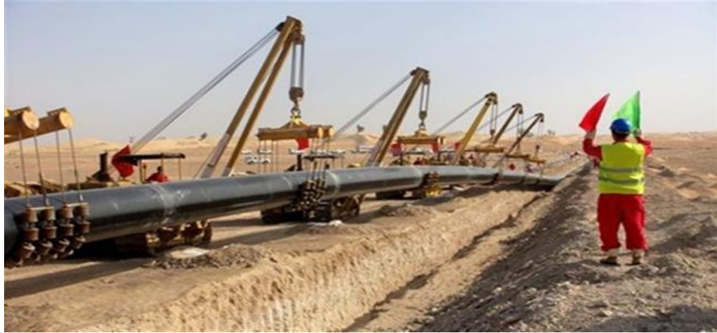
Fig A-13: A typical Pipeline construction activity
