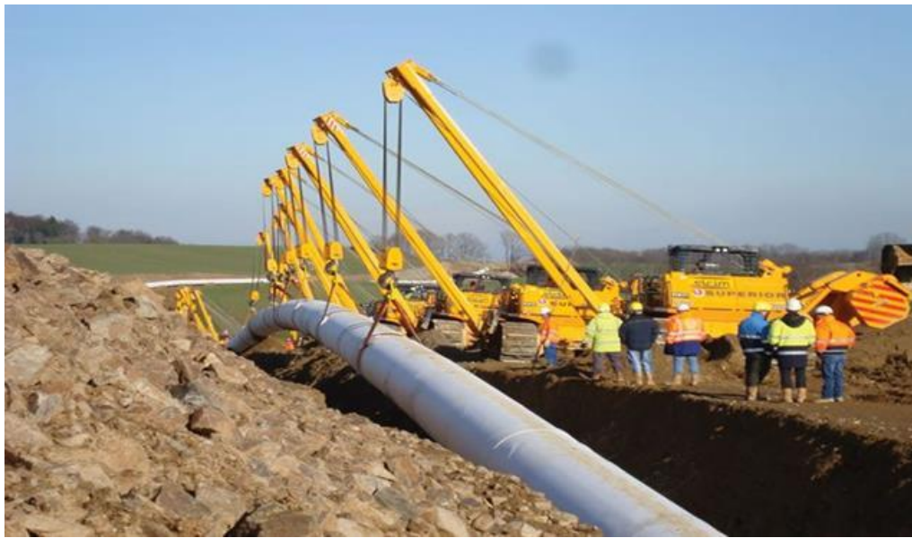
Fig A-12: A typical Pipeline construction activity
