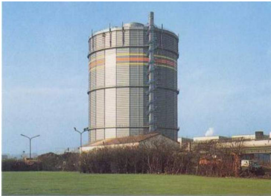
Fig 2.7 Leffer Waterless Gas holder
