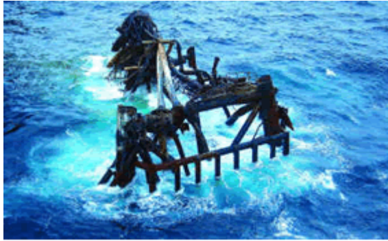
The MHN platform after collapse.
