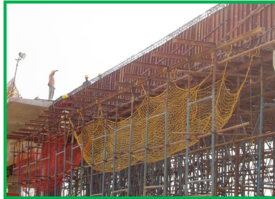
P-8: Safety Net used for height work
