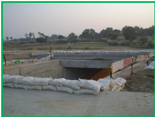
P-5: Gunny Bags barricading at Opening
