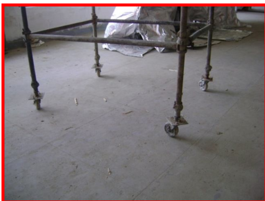
P-23: Rolling scaffolding without break
