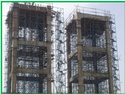
P-9: Safe Scaffolding
