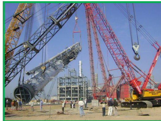
P-10: SOP followed for lifting of equipment
