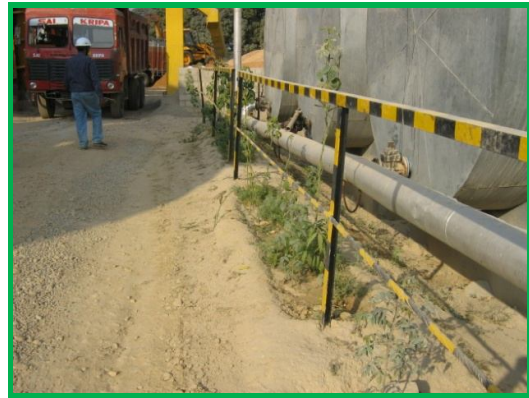
P-4: Hard Barricading at Hot Mix Plant
